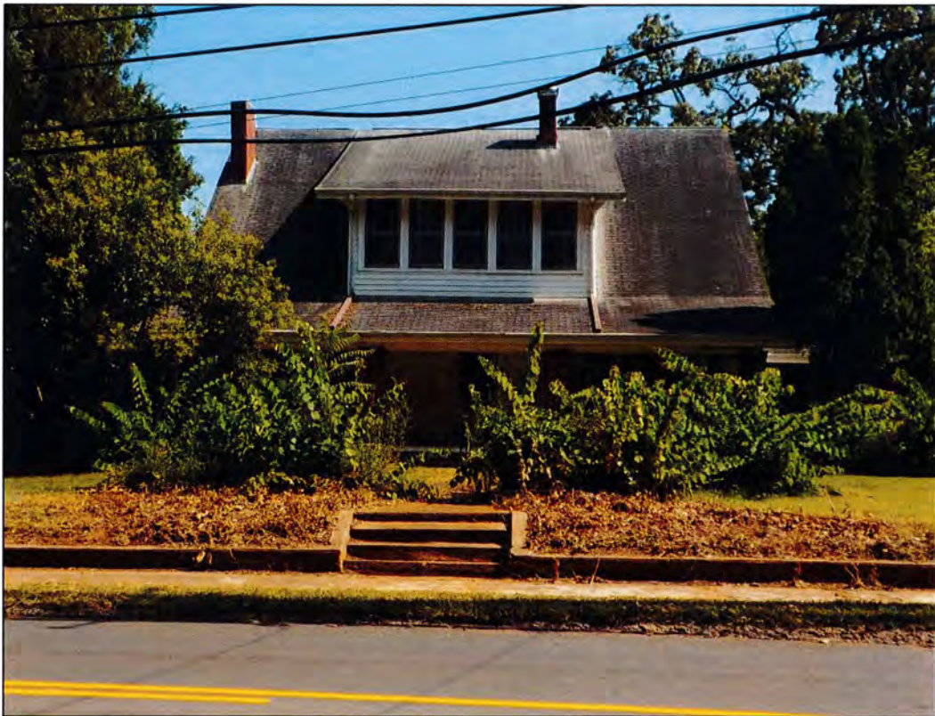
Figure 8. Structure CL1384, facing south.
