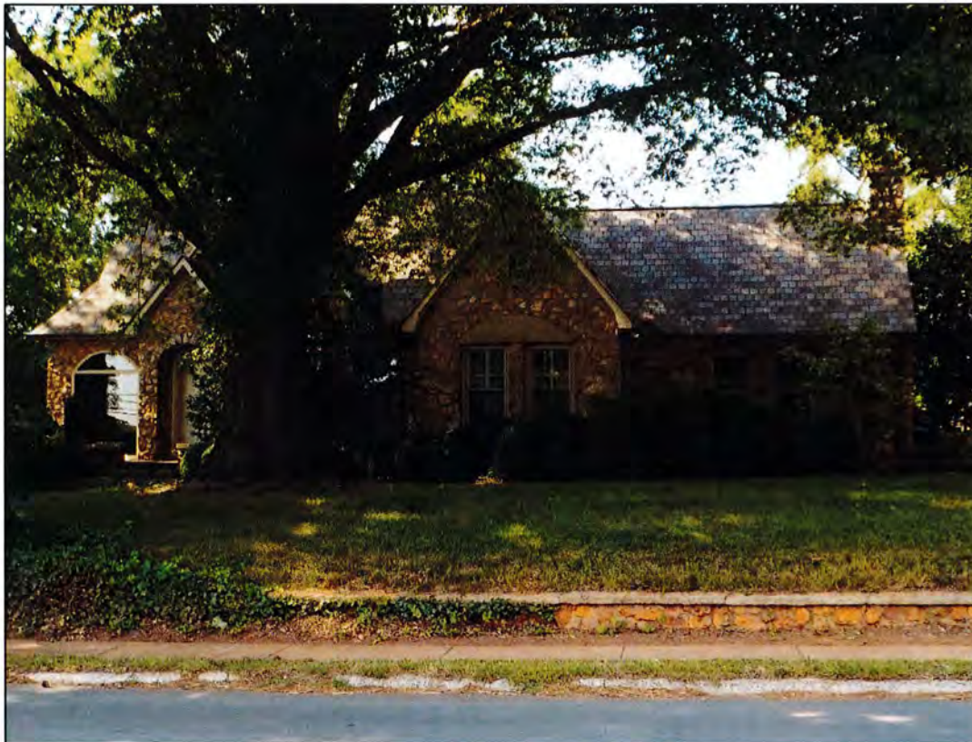
Figure 7. Structure CL1382, facing north.
